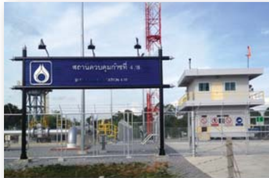
PTT BV STATIONS RAYONG - SARABURI
