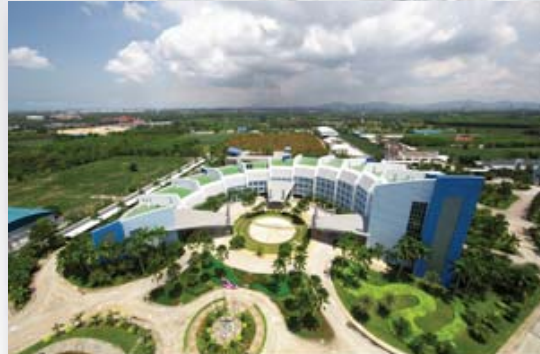
PTTGC OFFICE & TRAINING CENTER RAYONG
